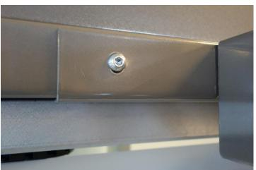
Close-up of one of the bolts fixing the leg section to the support structure.
